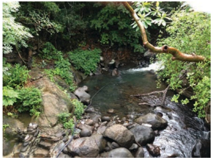
Riprapping with rocks keeps this stream from eroding the soil.
